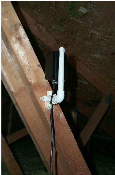
Here an antenna is mounted in an attic. PVC plumbing hardware is used to attach the antenna to the framing. The vertical pipe is not cemented to allow the antenna to be rotated slightly for fine-tuning direction. The front of the antenna must face exactly north.
